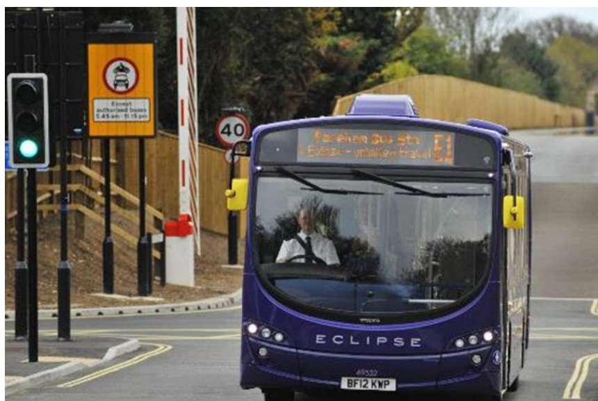
Figure 12 – The Fareham-Gosport BRT busway
